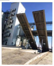
The Loading bins for trucks rest beside the workhouse building. The availability of passages in the upper side of the silo provides ease for workers to move , erect and check. BALAD AL-SILM ENGINEERING BUREAU
