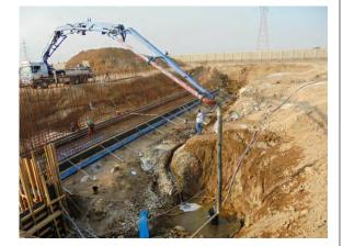
A reinforced concrete ring beam rest on piles will support 12 rectangular columns that in return will support a similar upper rectangular reinforced concrete beam that holds a concrete conical hopper of 10.35 m diameter
