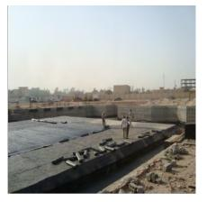
To avoid the high water table level in soil, the site was lifted by 90cm and a de watering process persisted during the substructure executing period. A huge concrete casting process (1700m3) for the raft beneath the diving pool and the basement was done. It took 16 hours for BALAD AL-SILM ENGINEERING BUREAU
