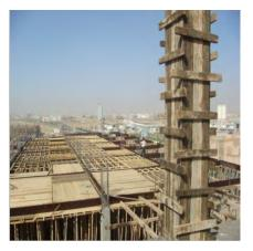
During the constructing of the ground floor columns a decision was made to reevaluate the weights and measurements of footings to see wether it is possible to put additional two stories and the results were good if we just enlarge the columns sizes and add few reinforcement bars to them.
