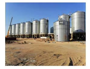
The bins are provided with emergency side discharge pipe and emergency access side wall door. The silo would be provided with passages ,stairs , to ease maintenance . BALAD AL-SILM ENGINEERING BUREAU
