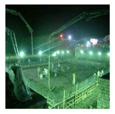
Several trial mix design jobs were done to reach the appropriate mix job with admixtures for 120 cm thickness raft cast in hot weather, intended to be impervious suitable for swimming pools. The raft Balad Al ilm included two parts with difference in finished level within 1.2 m thus we needed steel plate molds supported with bars to
